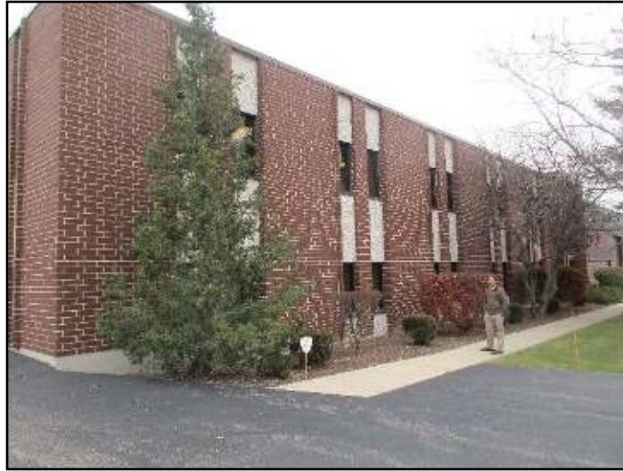
150. Concrete-block with brick-veneer
