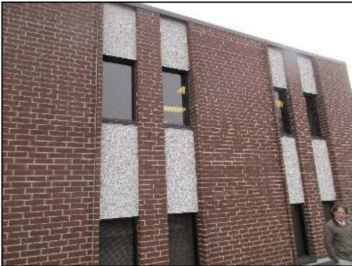
148. Concrete-block with brick-veneer
