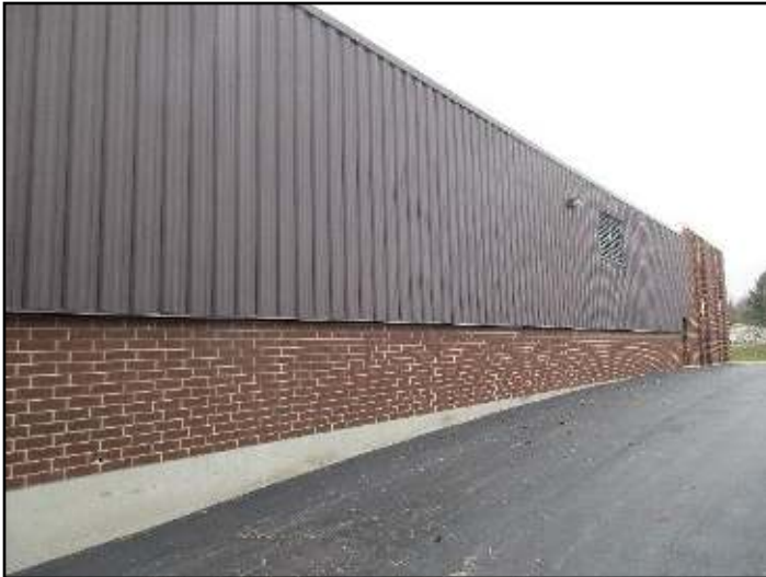
146. Concrete-block with brick-veneer
