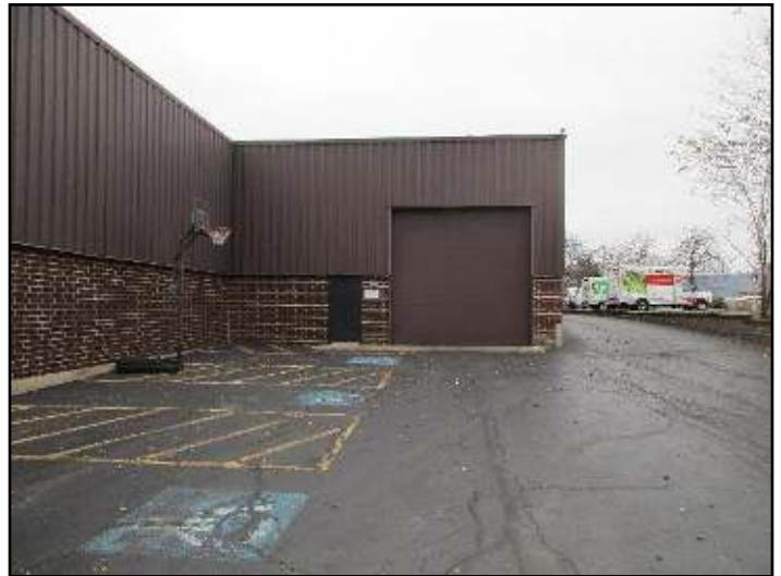
149. Concrete-block with brick-veneer
