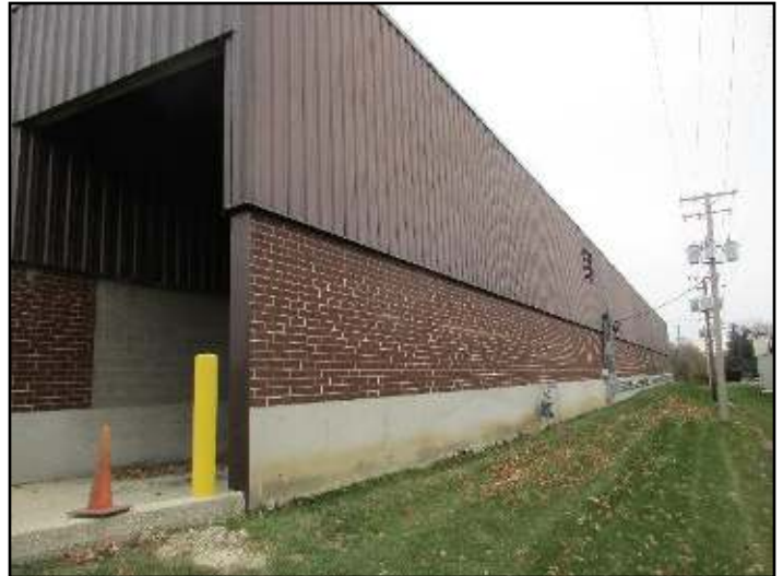
147. Concrete-block with brick-veneer
