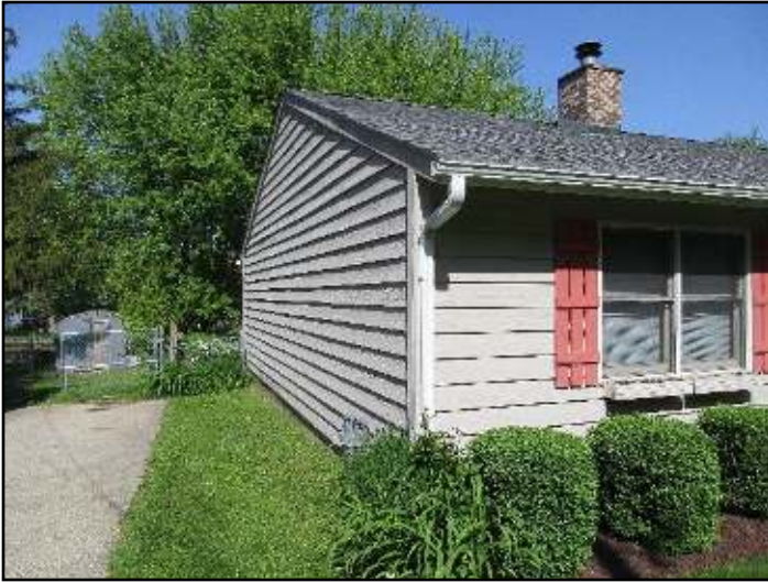
11. Hardboard, plywood or OSB
