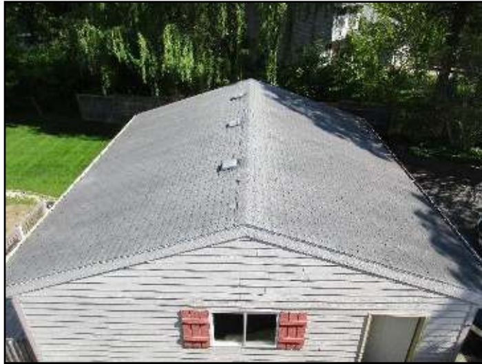
1. Asphalt shingles
