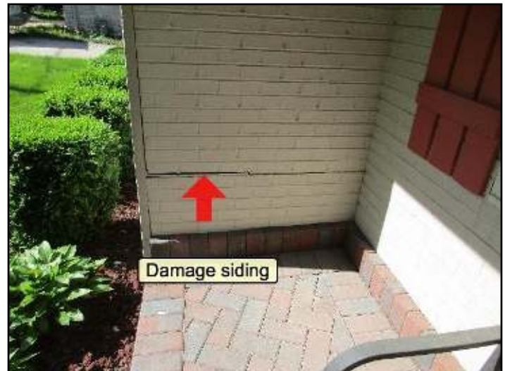
28. Mechanical damage
