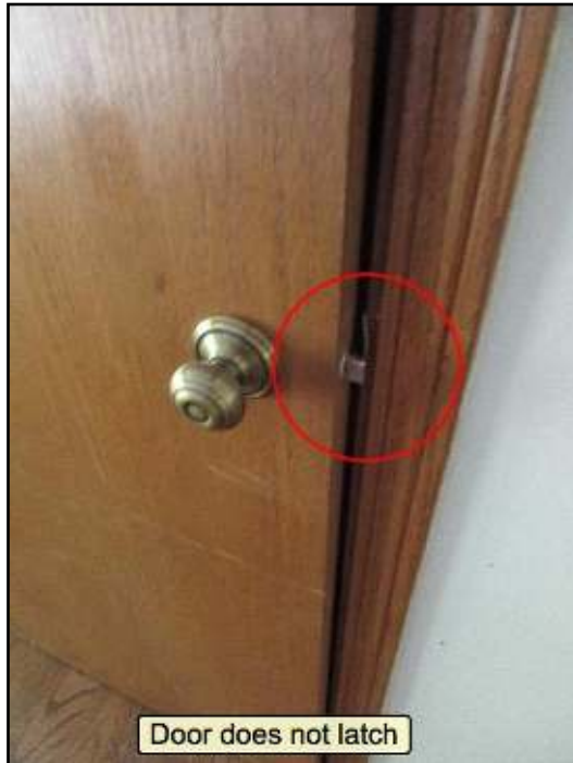
112. Loose or poor fit
