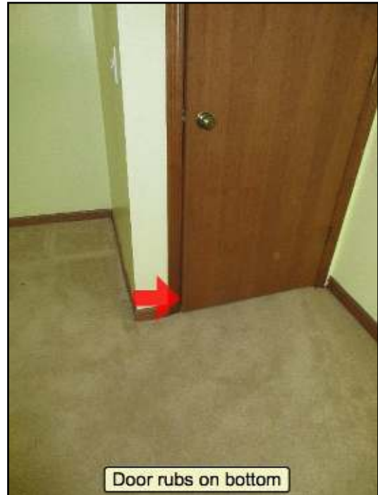
113. Loose or poor fit
